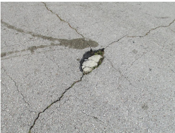
Asphalt pavement with pot hole
