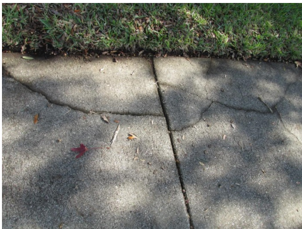
Concrete sidewalk with cracks
