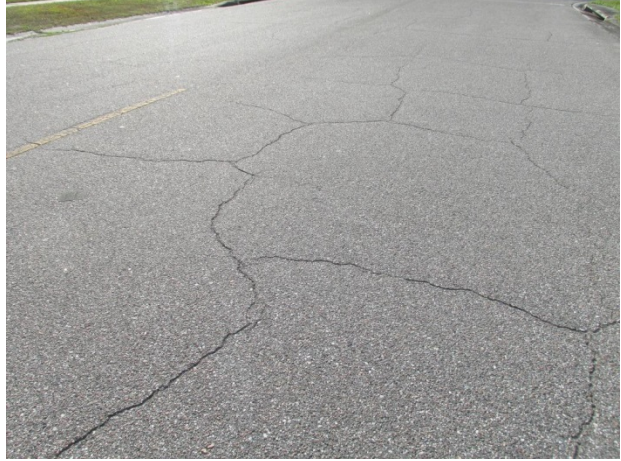
Asphalt pavement with block cracks
