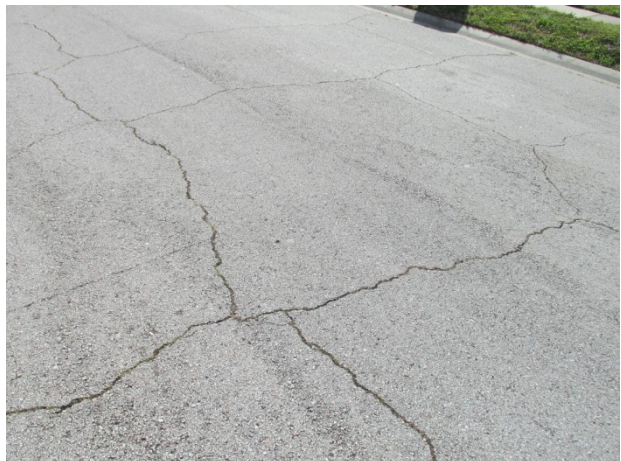
Asphalt pavement with block cracks
