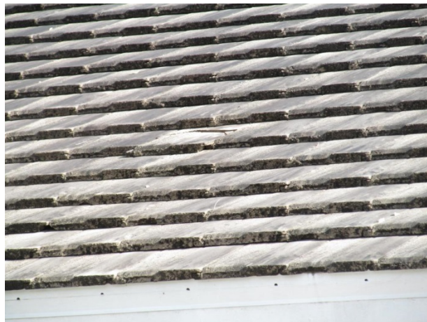
Concrete tile roof with broken tile
