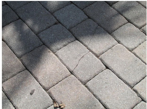
Masonry pavers with isolated cracks evident
