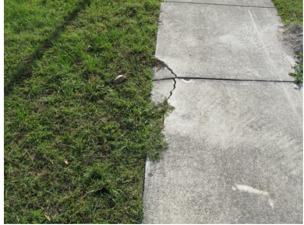
Concrete sidewalk with cracks
