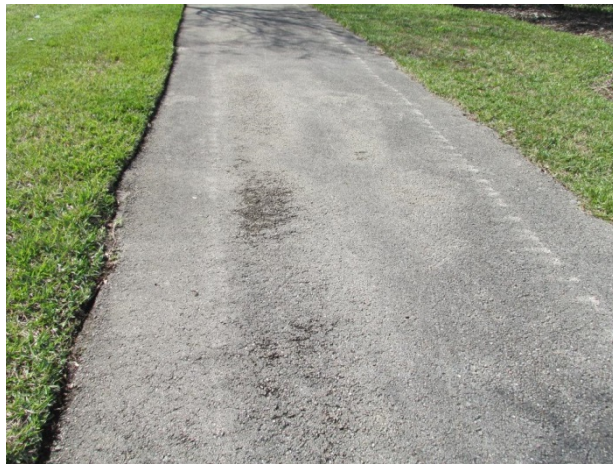
Asphalt walking path with surface deterioration
