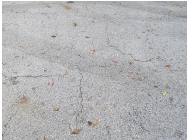
Asphalt pavement with alligator cracks
