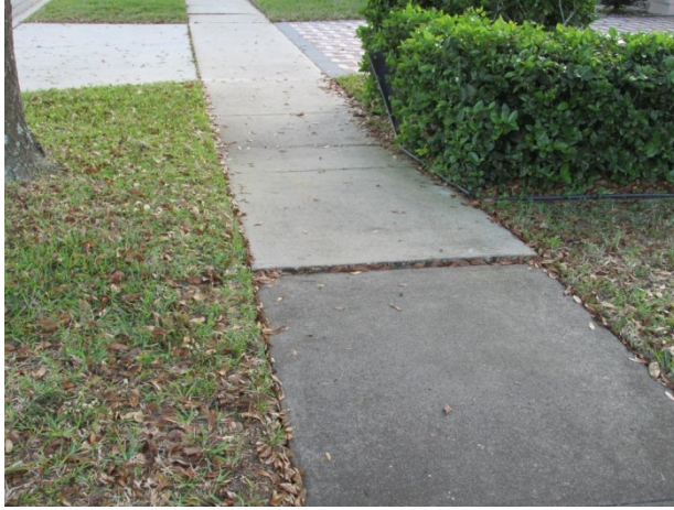
Concrete sidewalk with trip hazard
