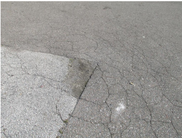
Asphalt pavement with alligator cracks
