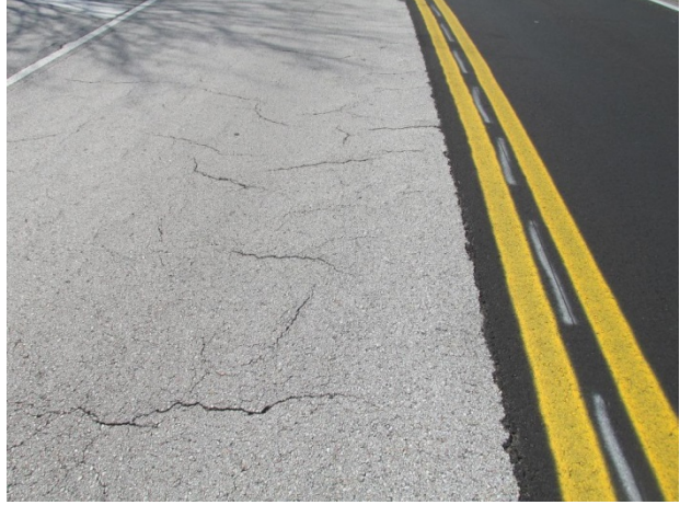
Asphalt pavement with slippage cracks
