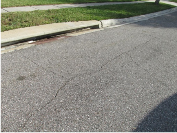
Asphalt pavement with block cracks
