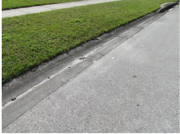
Concrete gutter with cracks
