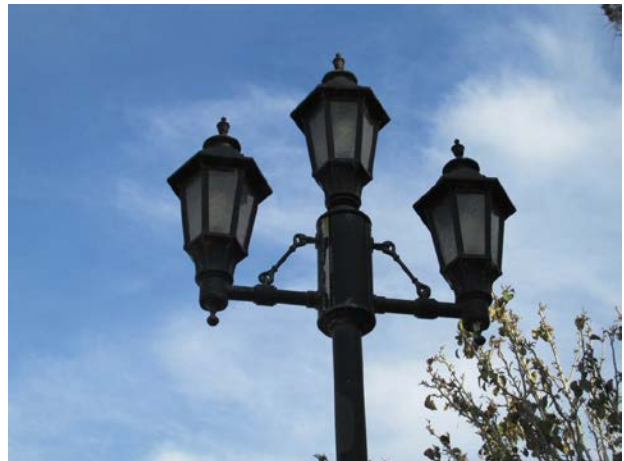
Finish deterioration at bridge light fixture
