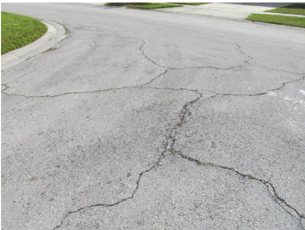
Asphalt pavement with block cracks
