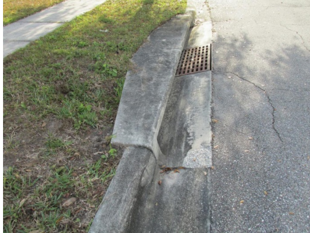
Severe settlement behind catch basin
