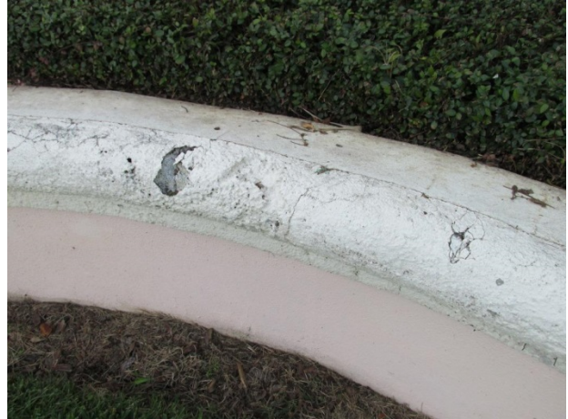
Coping damage at entrance signage
