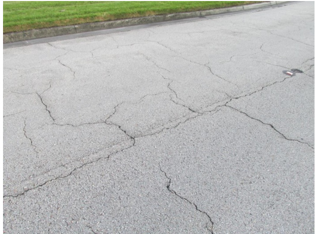
Asphalt pavement with severe block cracks
