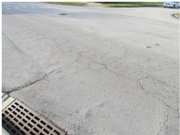
Asphalt pavement with alligator cracks and shoving
