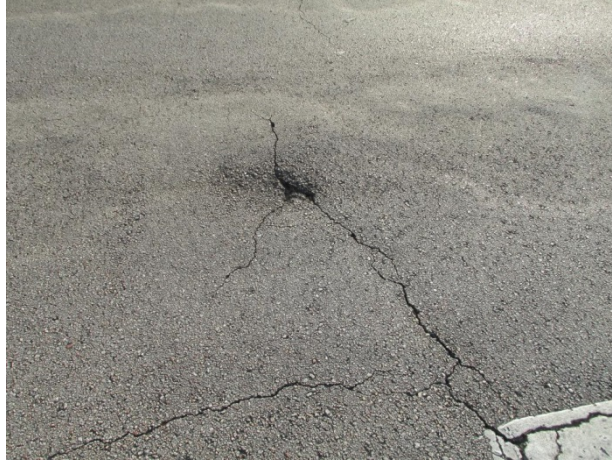
Asphalt pavement with pot hole
