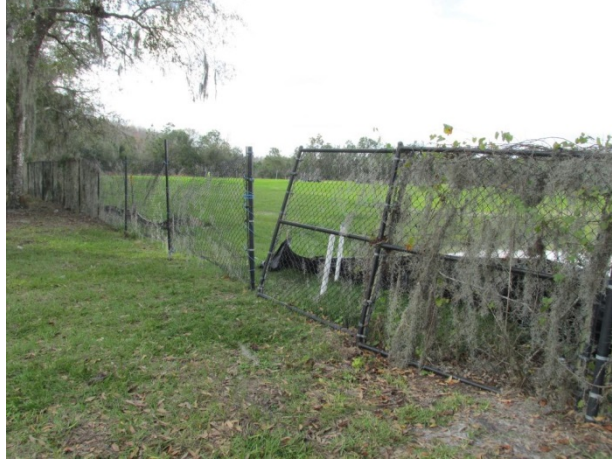
Chain link fence with lean evident
