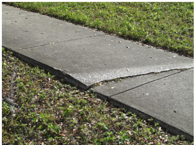
Concrete sidewalk with cracks and trip hazard
