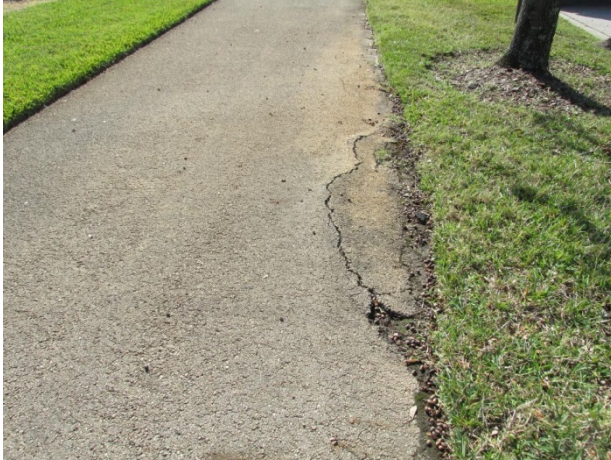
Asphalt pavement walkway with edge cracks
