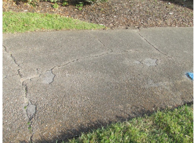
Asphalt pavement walkway with block cracks
