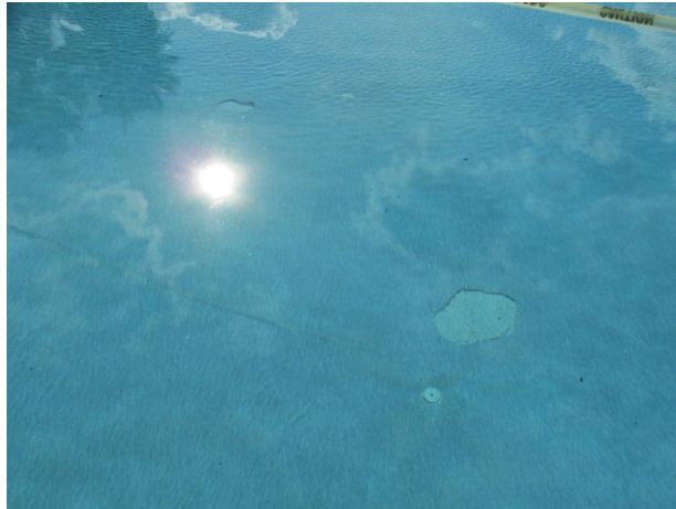
Missing plaster evident
