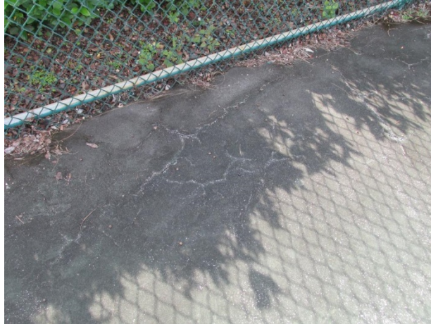
Hairline cracks evident
