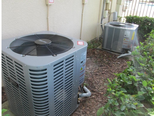
Condensing units for split systems
