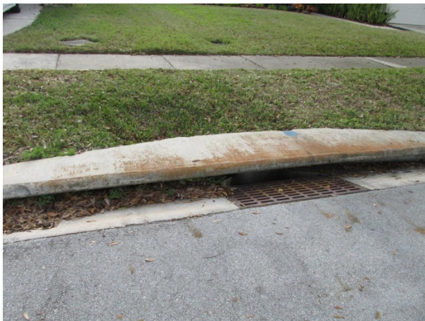
Severe settlement behind catch basin
