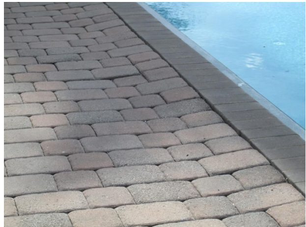
Deck pavers with isolated settlement evident
