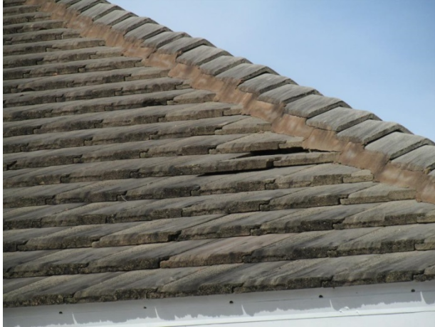
Concrete tile roof with loose tiles
