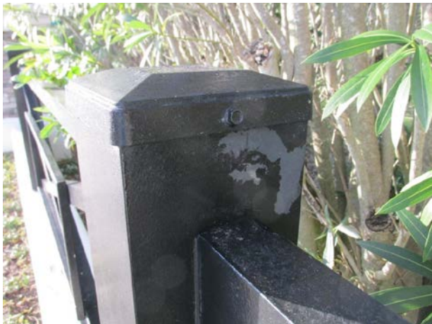
Finish deterioration at bridge railing
