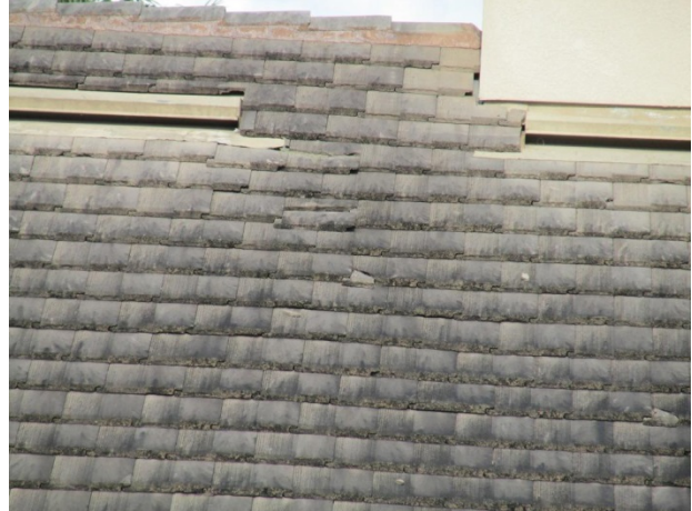
Concrete tile roof with broken tiles
