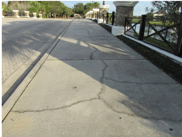
Concrete sidewalk with cracks
